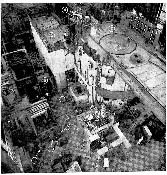
equipment will allow boiling-water and fog-cooling tests in the E-20 test-section by mid-1963. The J-16 loop being replaced by a new facility for materials testing in a high fast neutron flux, and a large organic-cooled loop will shortly be installed at the E-12 lattice site. Allowance for a loop in this position was included in the design of NRU some ten years ago.
